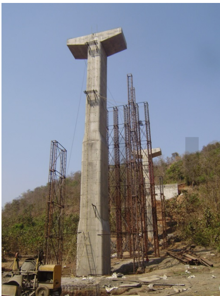
PHOTOGRAPH 5 PIER OF BRIDGE IN THANE DISTRICT
