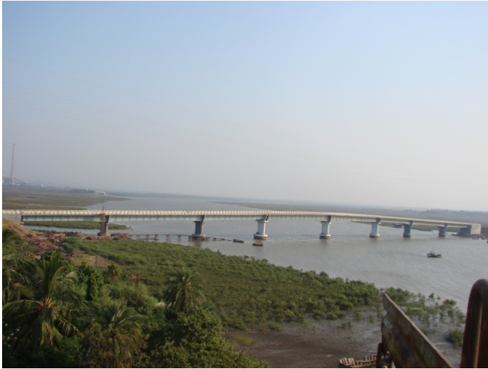
Photograph 2 DAHANU CREEK BRIDGE
