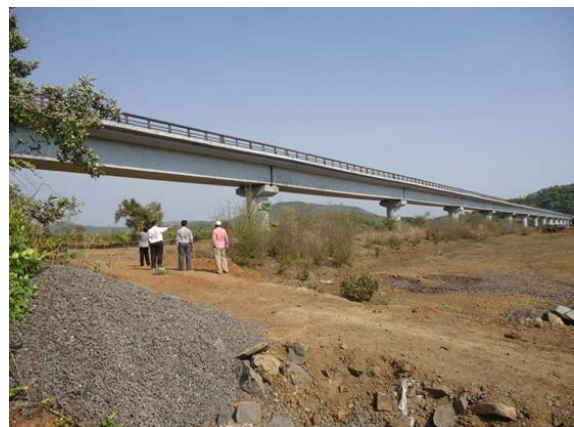
Photograph 1 MANDAD BRIDGE WITH R C C BOX SUPER STRUCTURE
